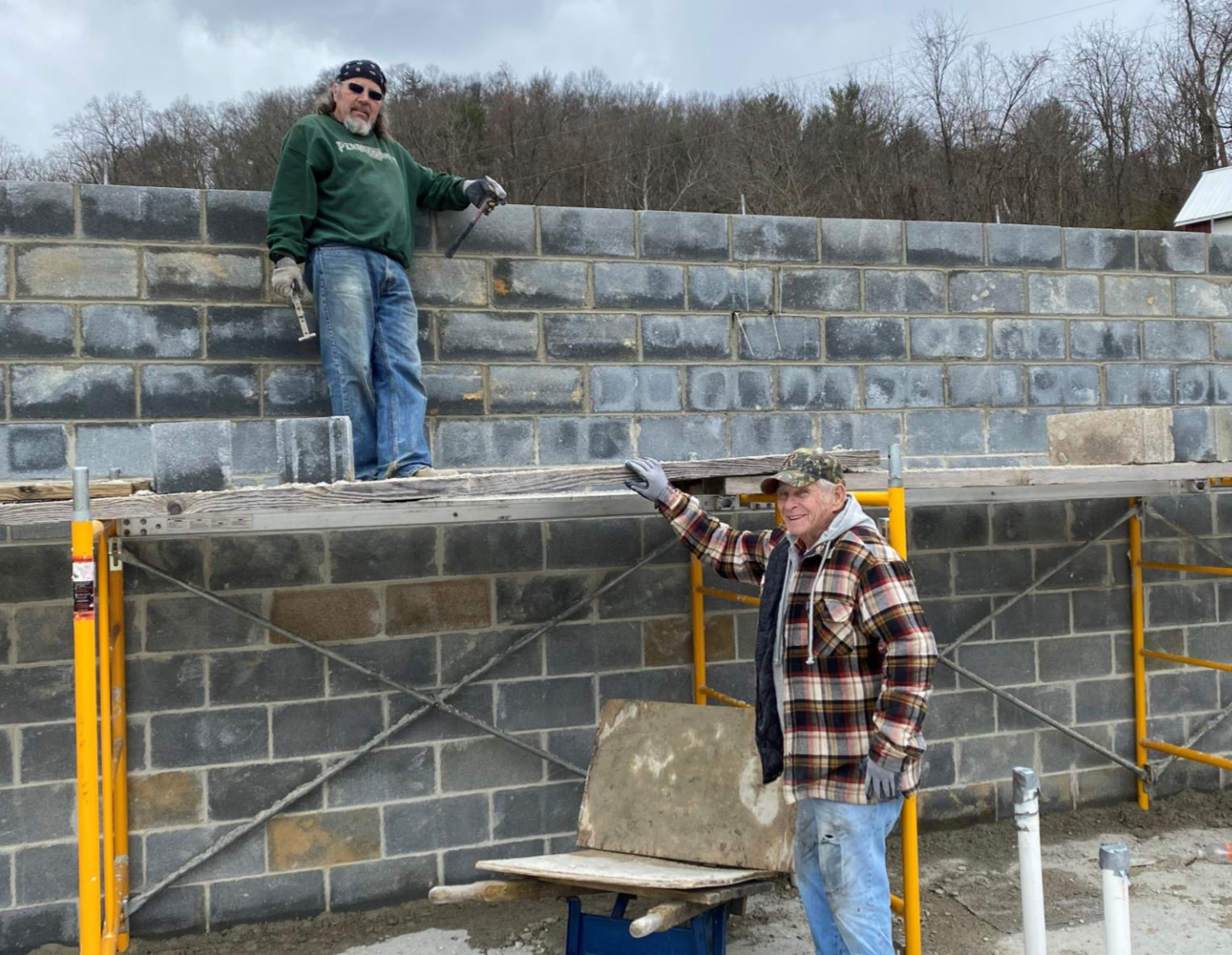
March 31 st (Actually April 1 st , but that is April fools day) -- Rich Morrow, George Pentz and Steve Steffel finish the bearing wall and seal up some wall sections under the windows and add insulation to the walls. Bond beam going in to the right.
