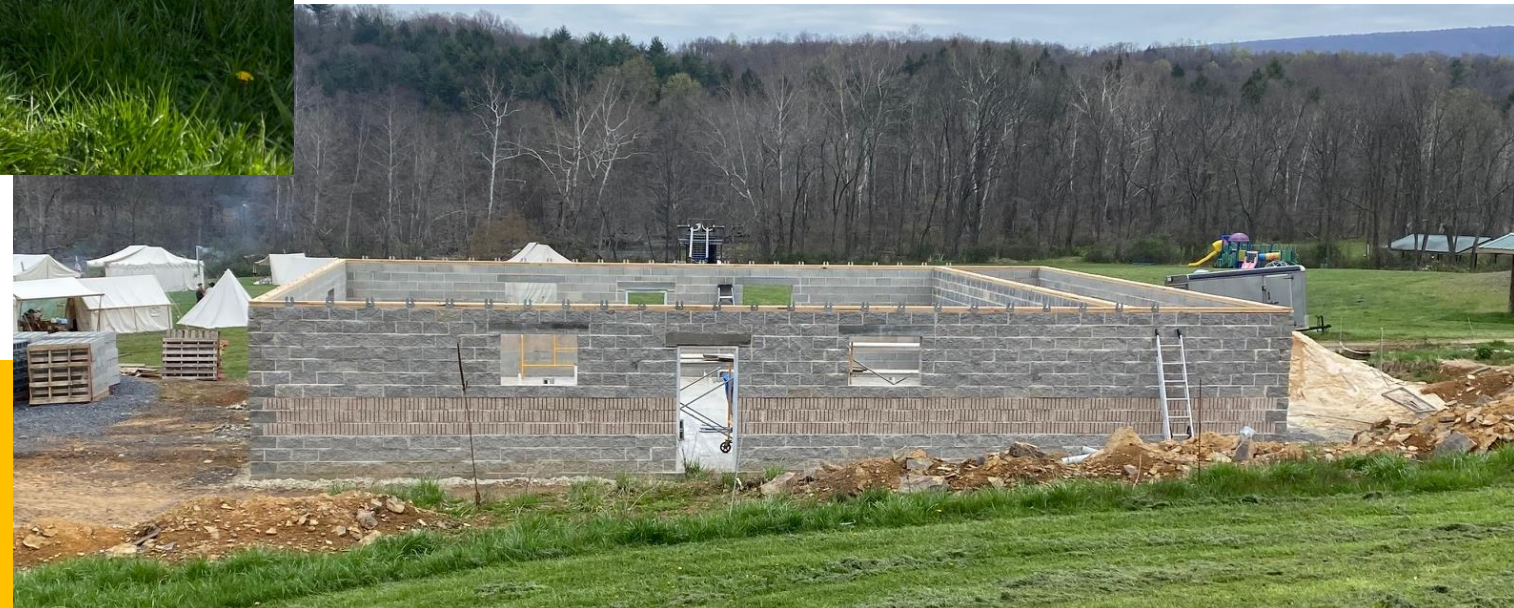
In April, George Pentz and Steve Steffel finished plates on top the wall and Steve added the hurricane ties to prepare for truss installation.
