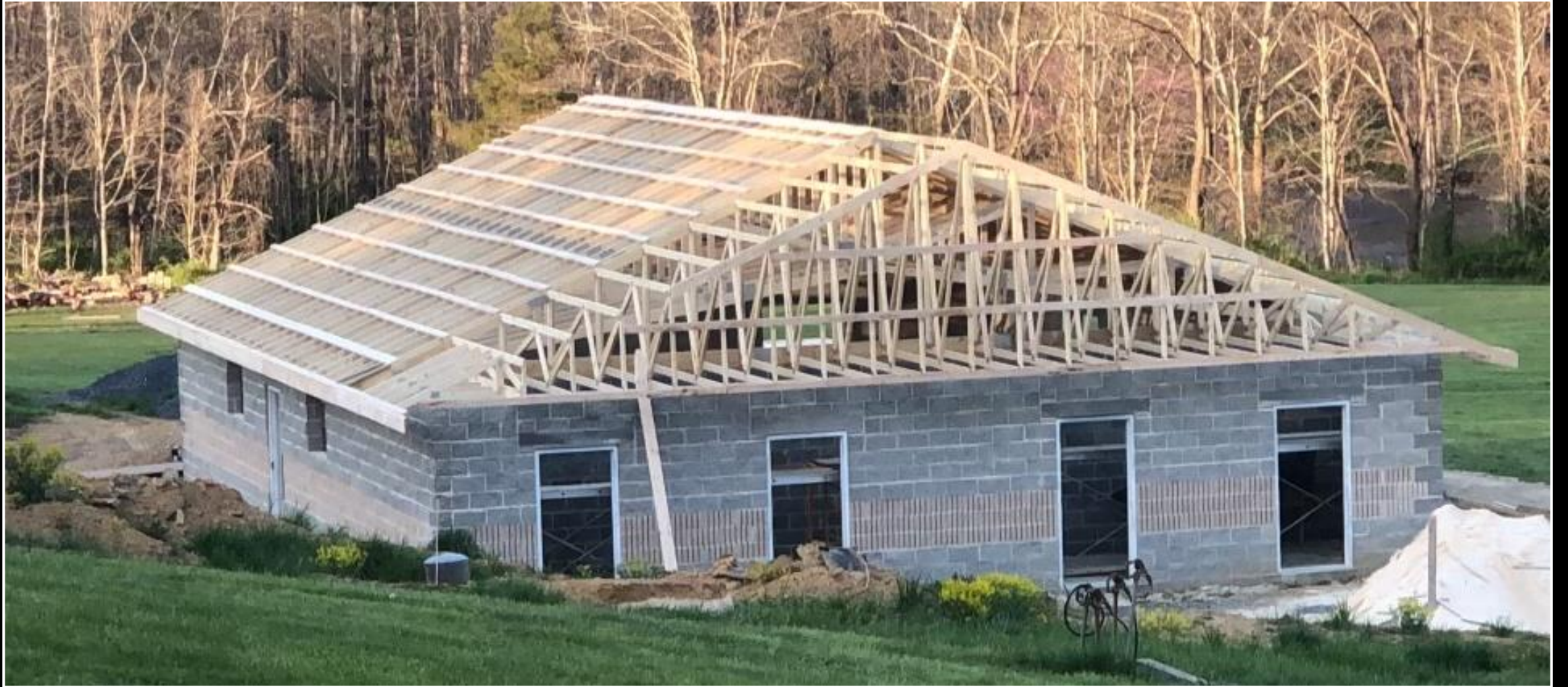
Trusses in place, a few more purlins needed – end of the day April 29
