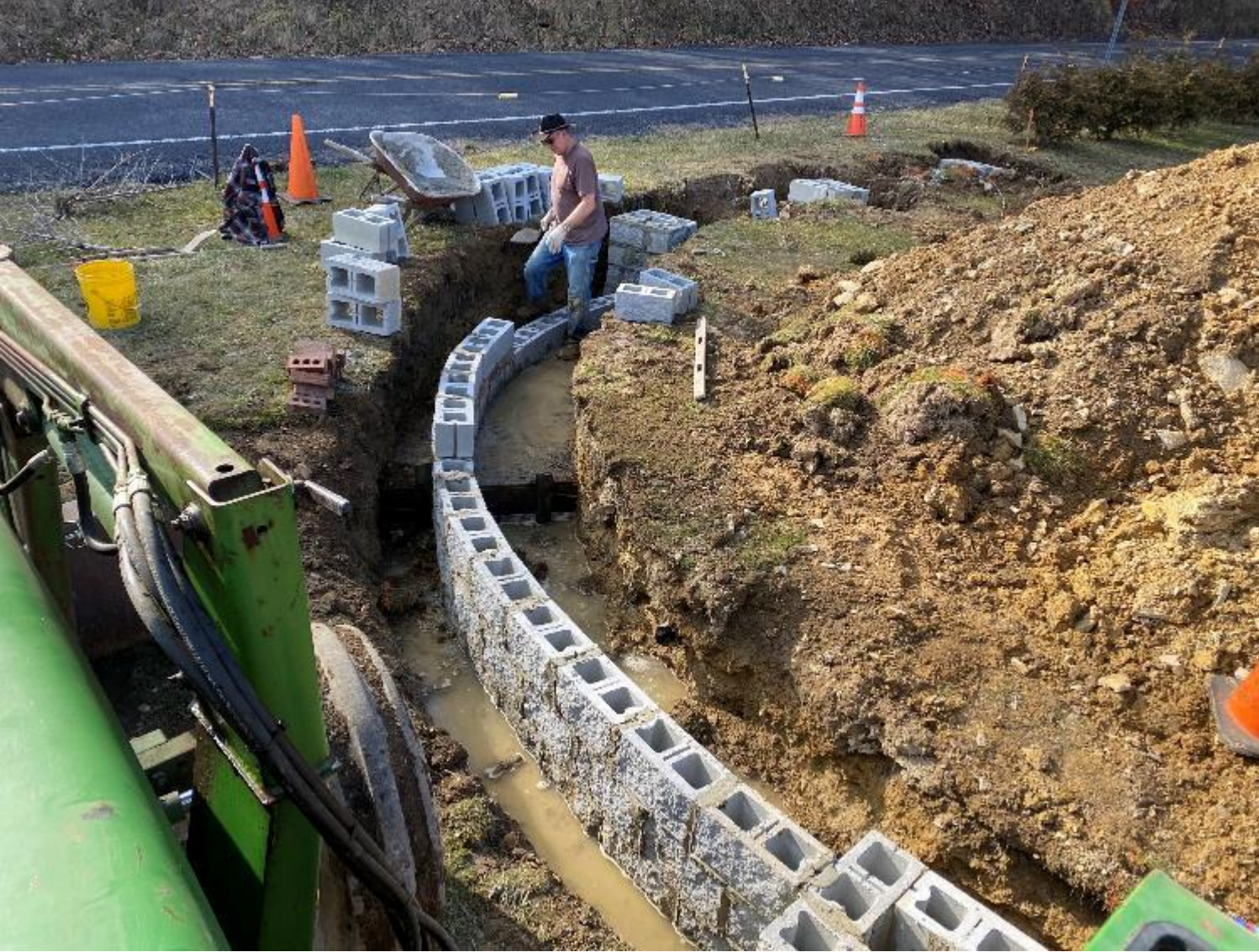
Feb 23, 2023 – Ron Adlesic and Steve work on the underground work for the decorative brick entrance wall - - almost a shame to cover it up - we are using left over split face block from the shower house. LanPro (Guy Jacobs our salesman) delivered the new 72" diesel zero turn, a ~30 year machine and in the evening, Scott Parthmore who had picked up the 15' batwing finish mower in NC brought it up to camp.
