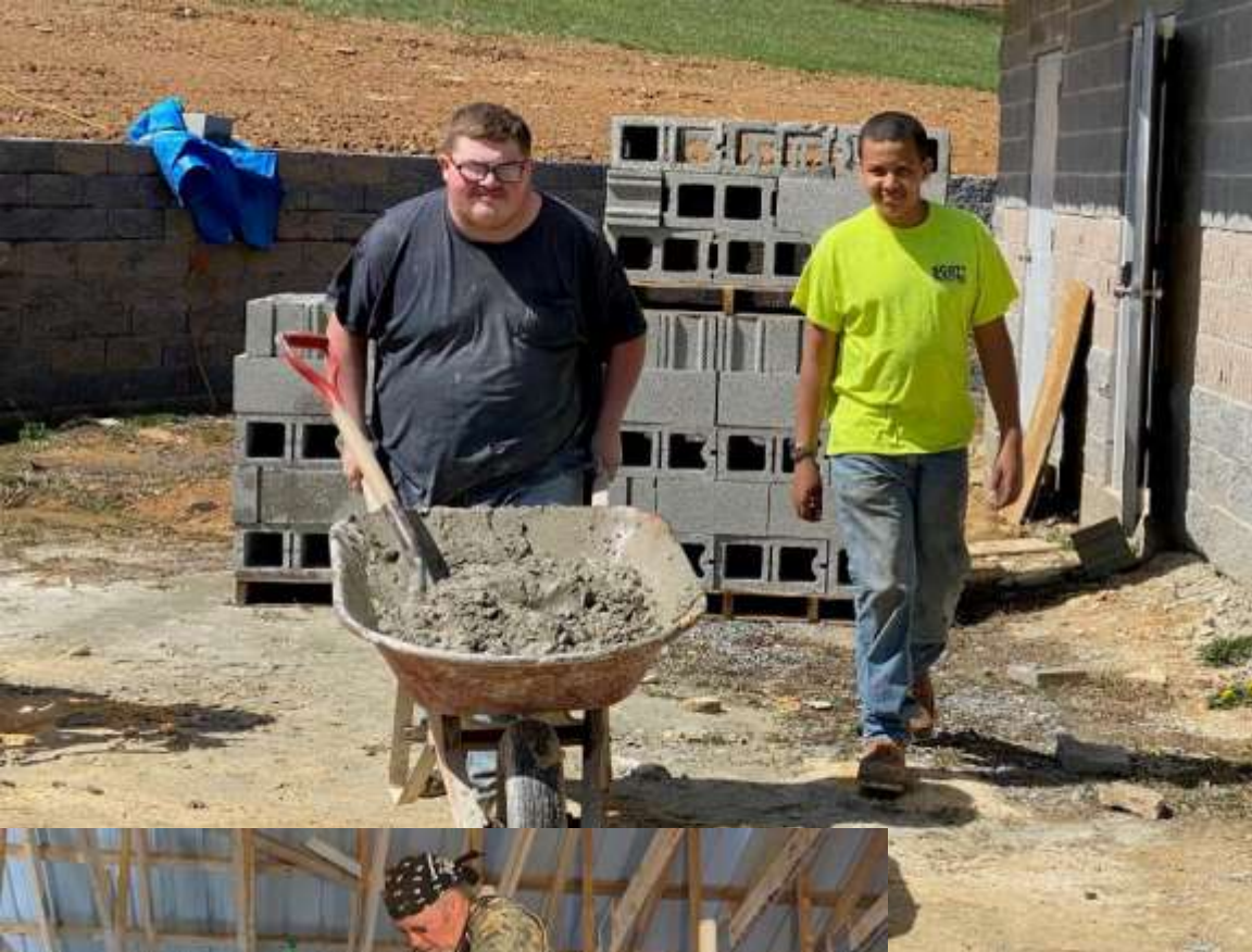
Rich Morrow and Brent Heller laying block between shower stalls.
