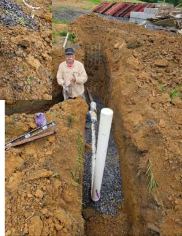
May 13 – Andy Baker, Mike Ardeno, George Pentz and Jadon Culp install 6” sewer line and two 1” electrical pipes to the back of the shower house where the septic tanks will be.
