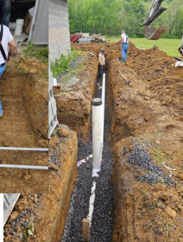
The pipe system includes a clean out, pipe for dump station and has capability of tying in future kitchen.
