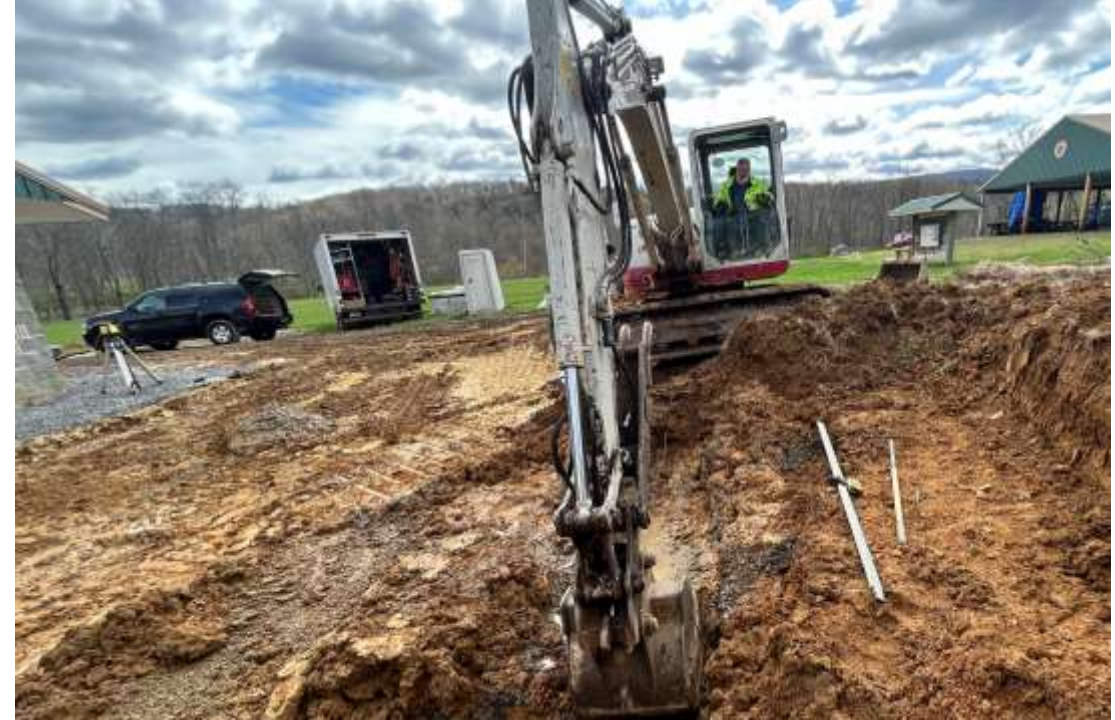
Andy Baker and Cord Hetrick getting ready to extend the retaining wall and then Cord and Andy install 2" pipe that will take liquids to the septic field up the hill.
